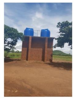
St. Lawrence water project included the drilling of the borehole, installing an electric water pump, building a pump house, installing a solar energy system connected with the electric pump, building a supporting frame holding two 5000-liter water tanks and installing an underground pipeline system. The work was implemented by Niho Systems from 4 November 2019 to 10 February 2020. The total amount of the project was **EUR 12,839.44**, which was equivalent to 10,464,143.60 Malawian Kwacha.
